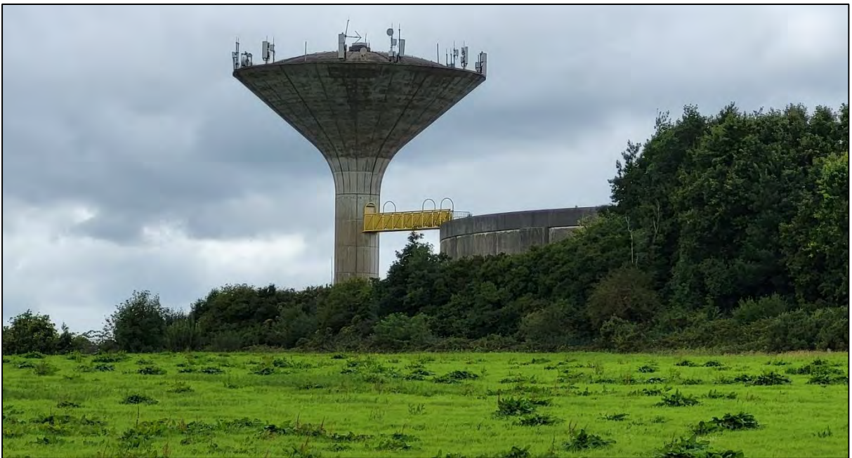
Plate 4: View of water tower and enclosed reservoir tank which are located adjoining the western site boundary.
